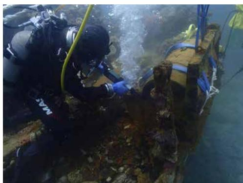
e. Removal work with an air saw
